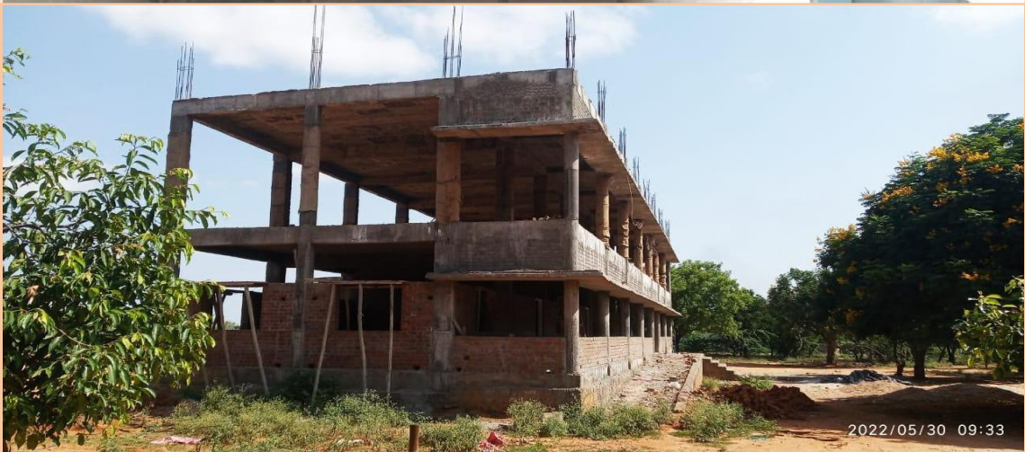
Construction of New Classrooms Block
